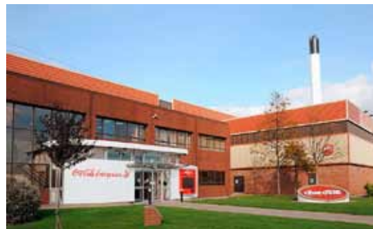
Coca-Cola's ISO 50001 certified facility in Wakefield, England, Europe's largest drinks manufacturing plant.
